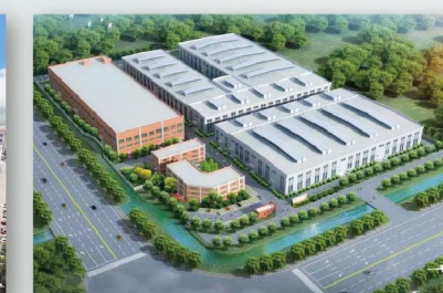
汉扬厂 Hanyang Factory
